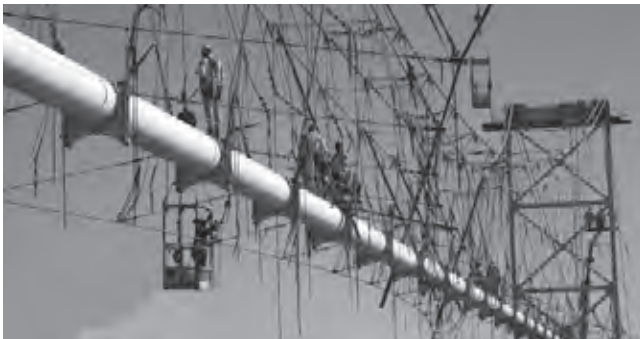
Williams Pipeline Bridge | Texas
