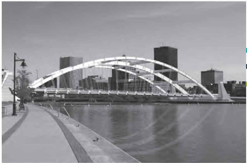
Troup-Howell Bridge | Rochester, NY
